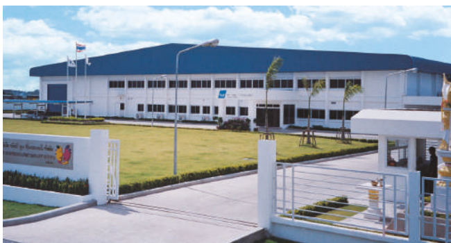
NT TOOL (THAILAND) CO., LTD. (OFFICE/FACTORY)
